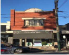
130 Burke Road, Malvern East
