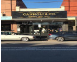
132 Burke Road, Malvern East
