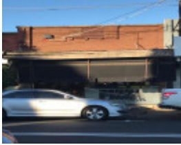
140 Burke Road, Malvern East
