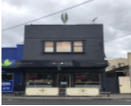
155 Burke Road, Malvern East
