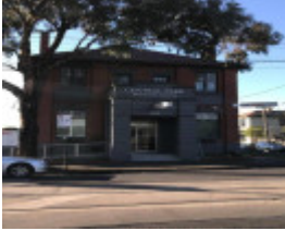
389 Wattletree Road, Malvern East
