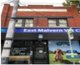
266 Waverley Road, Malvern East
