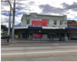
289 Waverley Road, Malvern East
