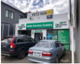
290 Waverley Road, Malvern East
