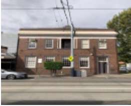
302-306 Waverley Road, Malvern East
