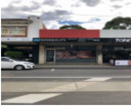
303 Waverley Road, Malvern East
