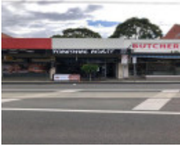
305 Waverley Road, Malvern East
