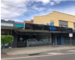
324 Waverley Road, Malvern East
