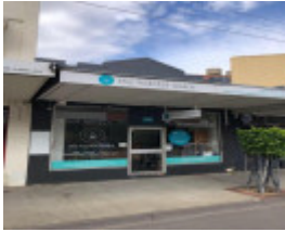
328 Waverley Road, Malvern East
