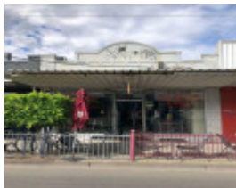
338 Waverley Road, Malvern East
