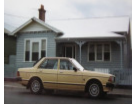
Source: GRS1160, Geelong Heritage Centre, c.1981 -85.
