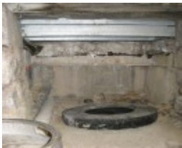
Oddfellows Hotel_Oct 2010_KJ_cellar_opening to Little Lonsdale now sealed
