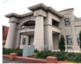
945-947 Dandenong Road, Malvern East
