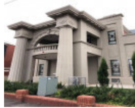
945-947 Dandenong Road, Malvern East
