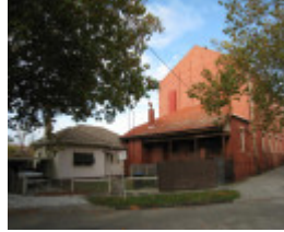
945-947 Dandenong Road, Malvern East
