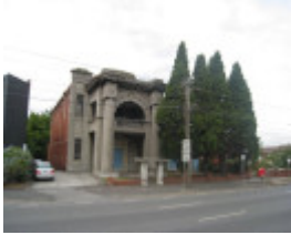
Former Morton Ray Masonic Temple Dandenong Road elevation.
