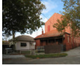
945-947 Dandenong Road, Malvern East
