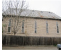
Spring Road hall.jpg (dem.2012)
