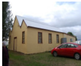
H2173 Black Lead Former Methodist Church and Hall 6
