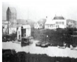
WEST BANK OF MOYNE RIVER, PORT FAIRY WHARF AND JETTY PRECINCT
