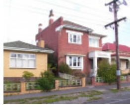
4A East Street South
