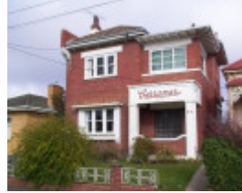
4A East Street South
