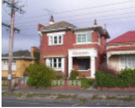
4A East Street South
