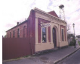
1 athenaeum library & town hall conness street chiltern front view
