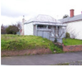
7 East Street South
