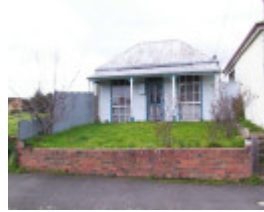
7 East Street South
