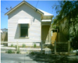
27 George Street, Geelong West
