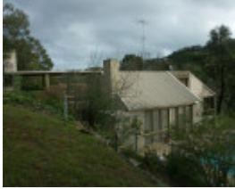
Residence, north and east elevations viewed from Jackman Rd
