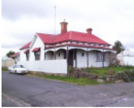
1 East Street South
