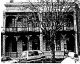
Terraces 30-32 Camp St - Ballarat Heritage Review, 1998
