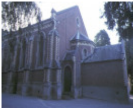
former congregational church brighton rear of church nov1984
