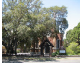
FORMER CONGREGATIONAL CHURCH SOHE 2008
