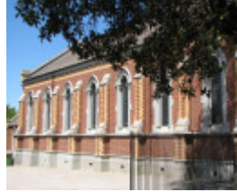
FORMER CONGREGATIONAL CHURCH SOHE 2008
