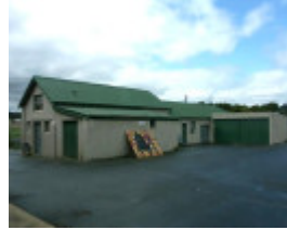
Building 3 Former Sloyd Room.jpg
