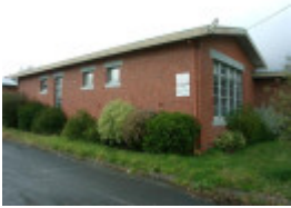
Building 4 Former Orphanage School.jpg
