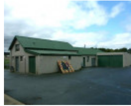
Building 3 Former Sloyd Room.jpg
