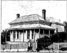
Darjeeling 6 Otway Street South - Ballarat Conservation Study 1978
