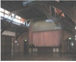
H0124 St Andrews Brighton Parish Hall interior May 2009
