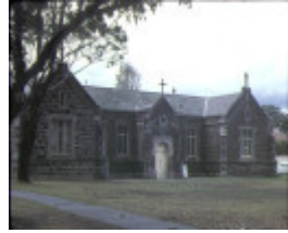
1 st andrews school house brighton front view
