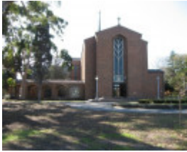
H0124 St Andrews Brighton church front elevation May 2009
