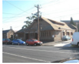
H0124 St Andrews Brighton Parish Hall exterior May 2009
