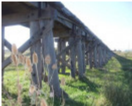
1604 Dennington Railway Bridge2
