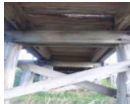
1604 Dennington Railway Bridge3
