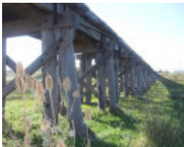
1604 Dennington Railway Bridge2
