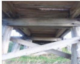
1604 Dennington Railway Bridge3
