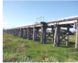
1604 Dennington Railway Bridge
