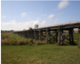
RAILWAY BRIDGE SOHE 2008
