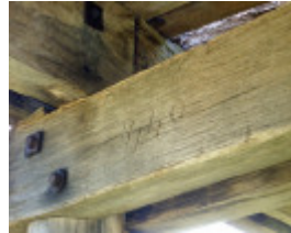
RAILWAY BRIDGE SOHE 2008
