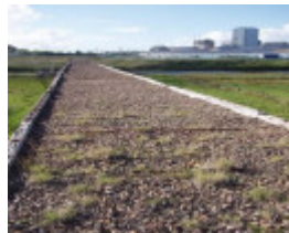
1604 Dennington Railway Bridge4
