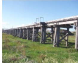
1604 Dennington Railway Bridge
