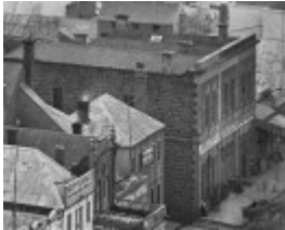
View of shops at 27, 29 & 31 Armstrong Street in 1873
