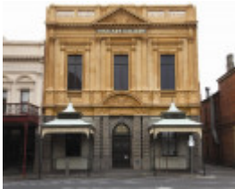
BALLARAT ART GALLERY_Restored Facade_Compressed.jpg 2010
