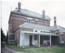
kiora south road brighton rear view nov1985
