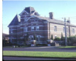
1 kiora south road brighton side view jun1981
