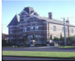
1 kiora south road brighton side view jun1981
