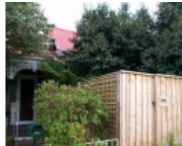
24 East Street South
