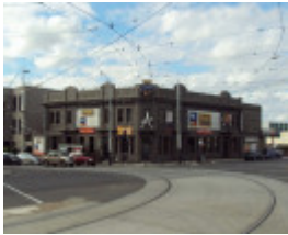
Former Railway Hotel
