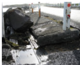
Warrnambool viaduct now_2009
