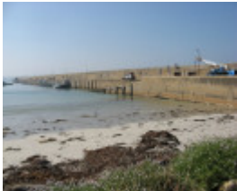
Warrnambool Concrete breakwater_KJ_May 09
