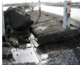
Warrnambool viaduct now_2009
