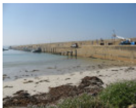
Warrnambool Concrete breakwater_KJ_May 09
