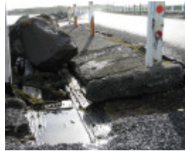
Warrnambool viaduct now_2009
