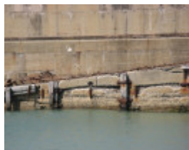
Warrnambool breakwater_ mass concrete_KJ_May 09
