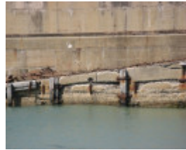
Warrnambool breakwater_ mass concrete_KJ_May 09
