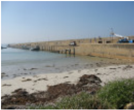
Warrnambool Concrete breakwater_KJ_May 09
