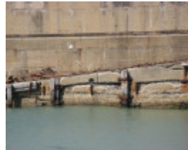
Warrnambool breakwater_ mass concrete_KJ_May 09
