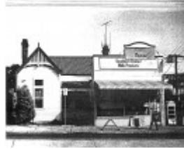
148 Mitchell Street: an altered but long term corner shop and residence which would have provided a focus for pre-car living in the precinct
