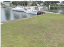
1026 - View of north portion of the site. Looking north west. (D. Tuck. 15/3/10)
