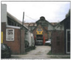
Photo 5: Section of original brewery building across Uley Street
