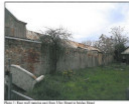
Photo 1: East wall facing west from Uley Street or bridge street.
