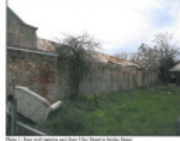
Photo 1: East wall facing west from Uley Street or bridge Street
