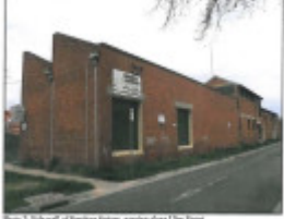
Photo 3: Side wall of former brewery building along Uley Street
