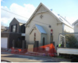
St James' Anglican Church (Former) 2012
