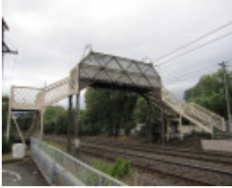
Railway Place West, Predestrian Bridge.JPG
