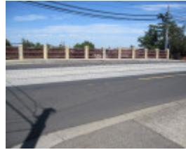
Maribyrnong Road Bridge
