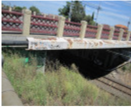
Maribyrnong Road Bridge
