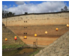
The inner face of the Lower Stony Creek Dam Wall showing some water in the reservoir.jpg
