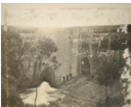
The outer face of the Lower Stony Creek Dam Wall c.1910 Image Geelong Heritage Service.jpg
