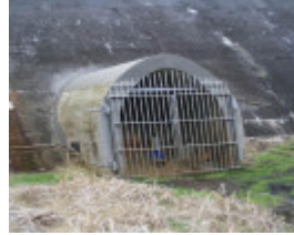
The western valve house.jpg
