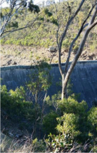
Lower Stony Creek Dam Wall.jpg
