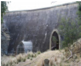
The Valve Houses (The left one is the West Valve House).jpg
