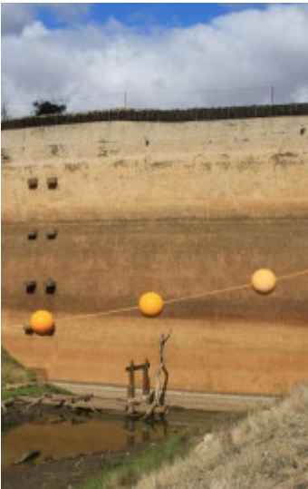
The inner face of the Lower Stony Creek Dam Wall showing some water in the reservoir.jpg
