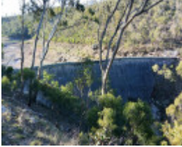
Lower Stony Creek Dam Wall.jpg
