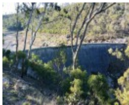
Lower Stony Creek Dam Wall.jpg
