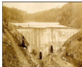
The outer face of the dam wall during construction 1873 (Image Barwon Water).gif
