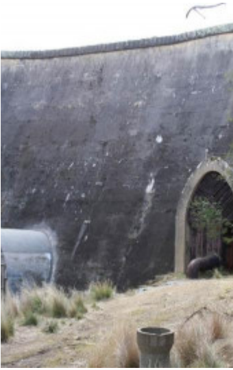
The Valve Houses (The left one is the West Valve House).jpg
