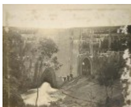
The outer face of the Lower Stony Creek Dam Wall c.1910 Image Geelong Heritage Service.jpg
