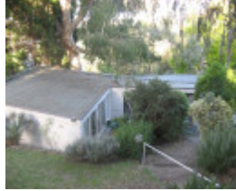
Snelleman House former carport
