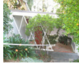
Snelleman House entrance porch
