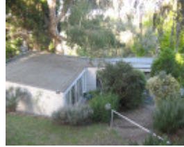
Snelleman House former carport
