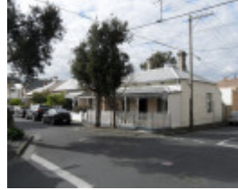
Lyndhurst Street, east side, north of Abinger Street
