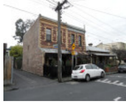
Two storey bi-chrome brick houses at 23 & 25, and house 27 Abinger Street
