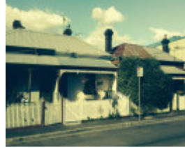
Attached cottages with shared roofs, 35-41 Glass St
