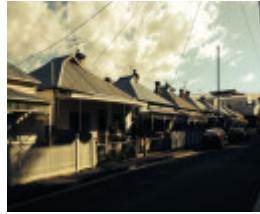
Similarly styled Edwardian timber houses at 6, 8 & 12-20 Stawell St
