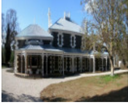
Eynesbury Homestead - Eynesbury Road EYNESBURY, MELTON SHIRE
