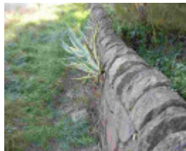
Dry Stone Wall M176 - HaHa Wall
