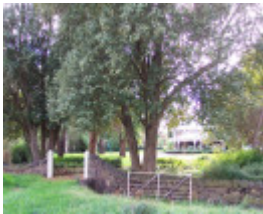
Dry Stone Wall M176 - HaHa Wall
