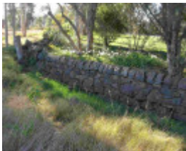
Dry Stone Wall M176 - HaHa Wall
