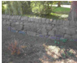
Dry Stone Wall M176 - HaHa Wall
