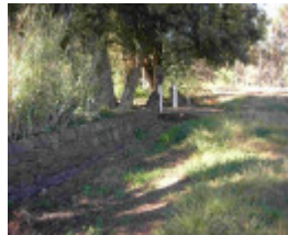
Dry Stone Wall M176 - HaHa Wall
