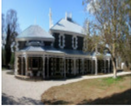
Eynesbury Homestead - Eynesbury Road EYNESBURY, MELTON SHIRE
