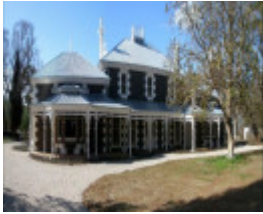
Eynesbury Homestead - Eynesbury Road EYNESBURY, MELTON SHIRE
