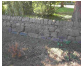
Dry Stone Wall M176 - HaHa Wall
