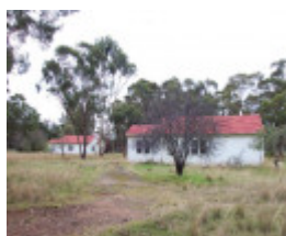
Prefabricated Myer houses
